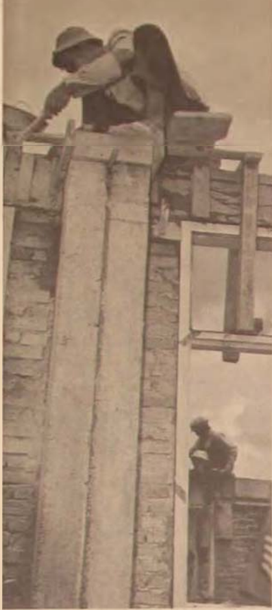
Vietnamese workers complete the brick understructure of a masonry barracks.
